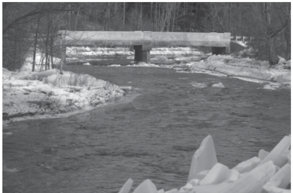
VTrans recently completed its East Corinth Bridge project. Total Cost: Approximately $745,000
