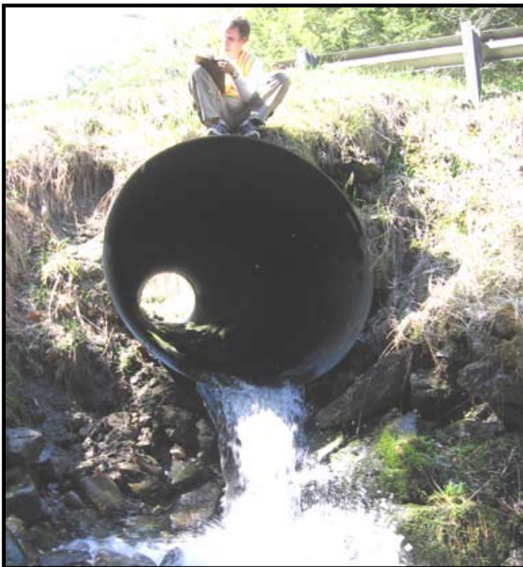
Pete Fellows collecting culvert data
