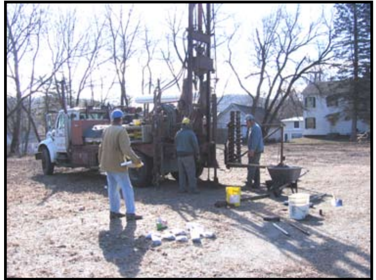
Groundwater Monitoring Wells going in at the Tip Top Tire site
