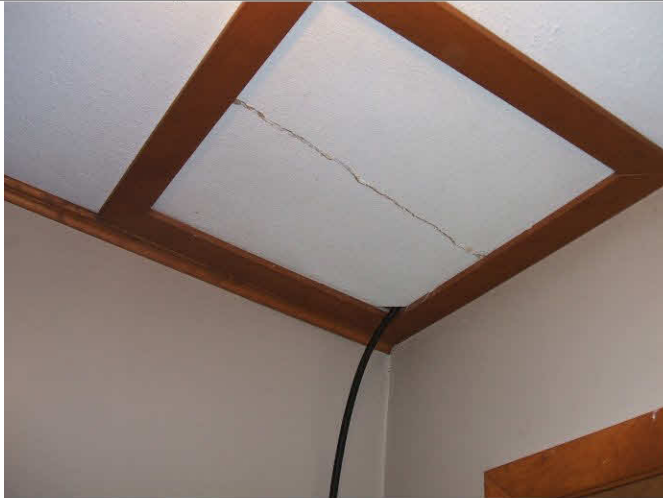
Broken attic hatch
