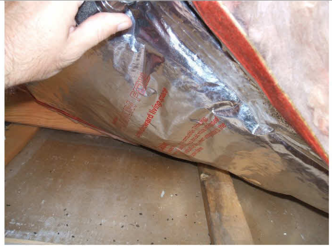
Attic insulation with strapping below
