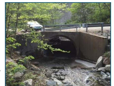
The Churchville Road culvert that will be replaced with CDBG-DR funds.
