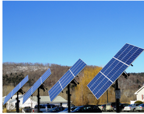
Tracking solar array | © Green Energy Times
