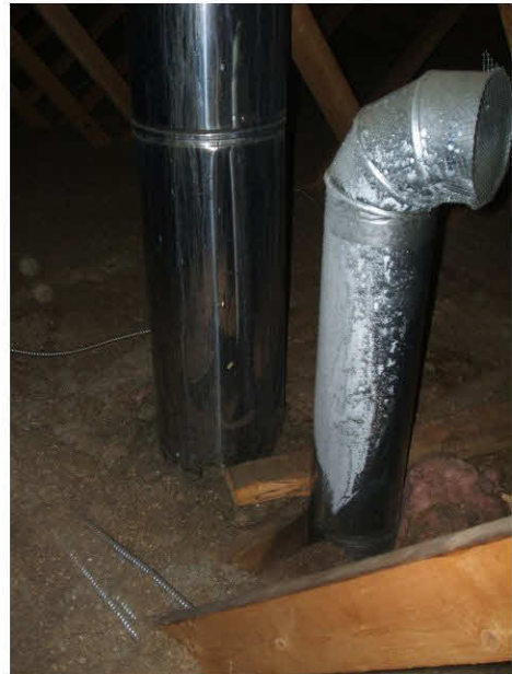
Similar to the truss brace above, warm air is keeping the bottom of this intake pipe warm and depositing frost on the cooler part above. This pipe needs to be foam sealed at the sheetrock.
