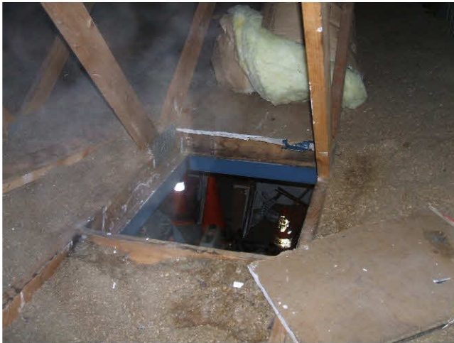
The attic hatch is a panel of broken sheetrock.
