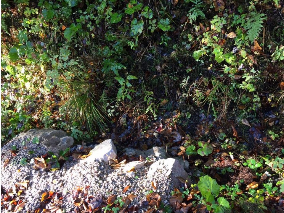
Culvert 2 inlet. Photo taken by TRORC staff.
