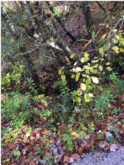
Culvert 2 outlet I. Photo taken by TRORC
