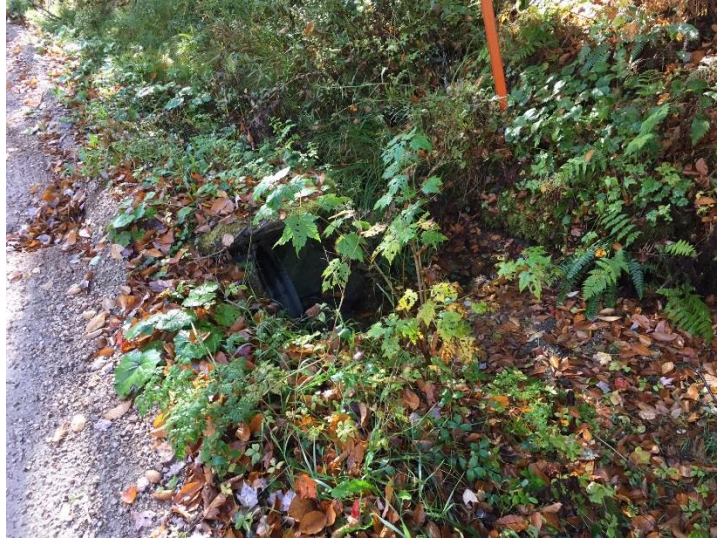
Culvert 2 inlet. Photo taken by TRORC staff.
