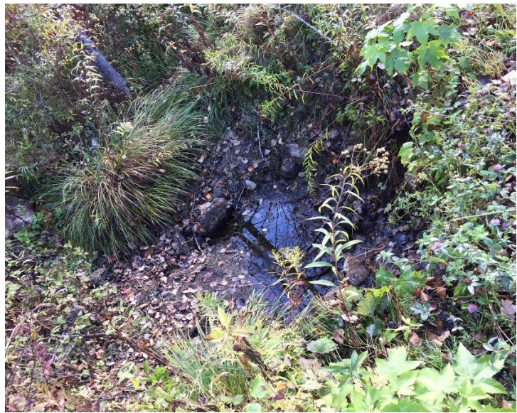
Culvert 1 outlet. Photo taken by TRORC staff.
