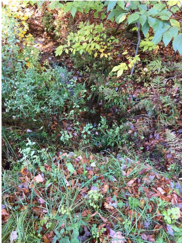
Culvert inlet. Photo taken by TRORC staff.
