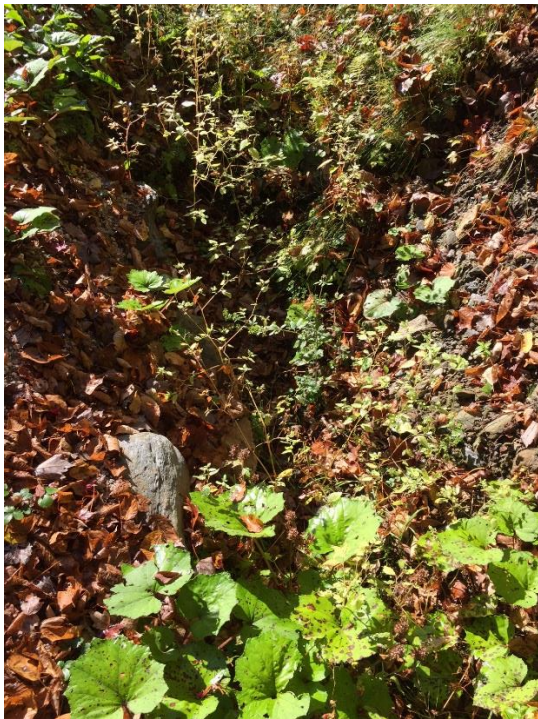
Culvert 1 inlet. Photo taken by TRORC staff.
