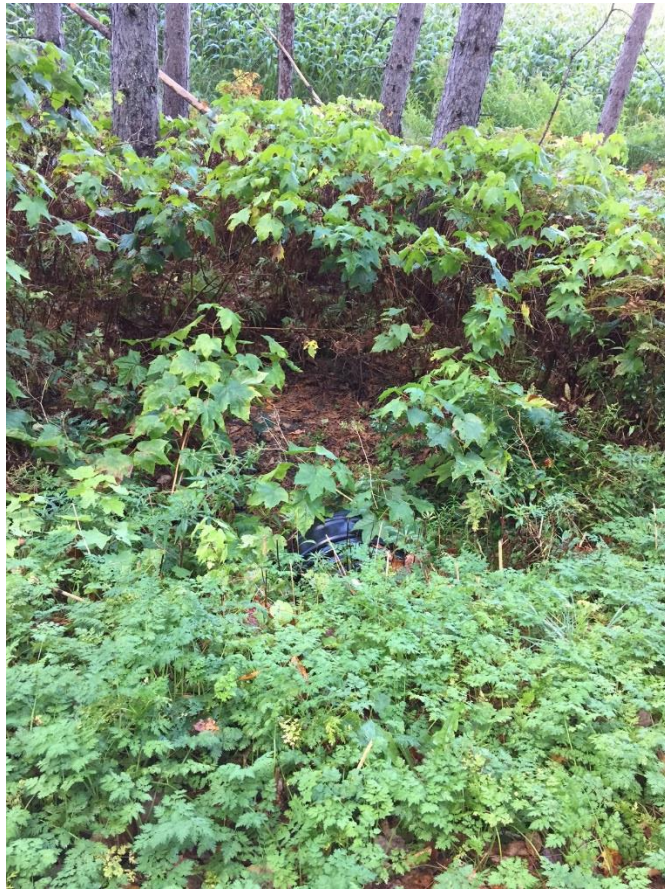
Culvert outlet. Photo taken by TRORC staff.
