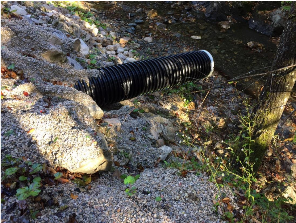
Culvert 2 outlet. Photo taken by TRORC staff.
