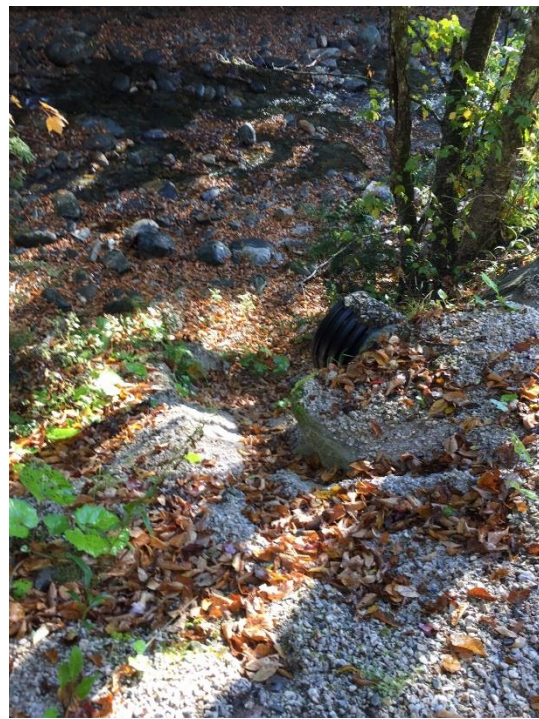
Culvert 1 outlet. Photo taken by TRORC staff.
