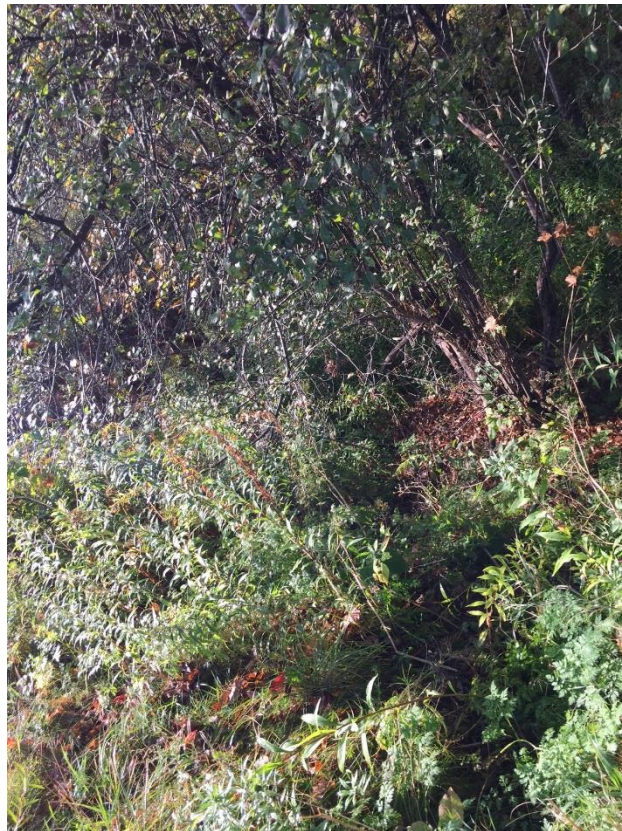
Culvert outlet. Photo taken by TRORC staff.
