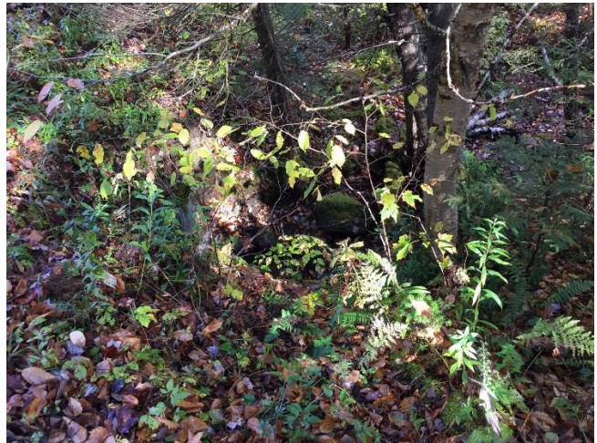
Culvert 2 outlet II. Photo taken by TRORC staff.
