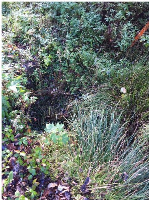
Culvert 1 inlet. Photo taken by TRORC staff.
