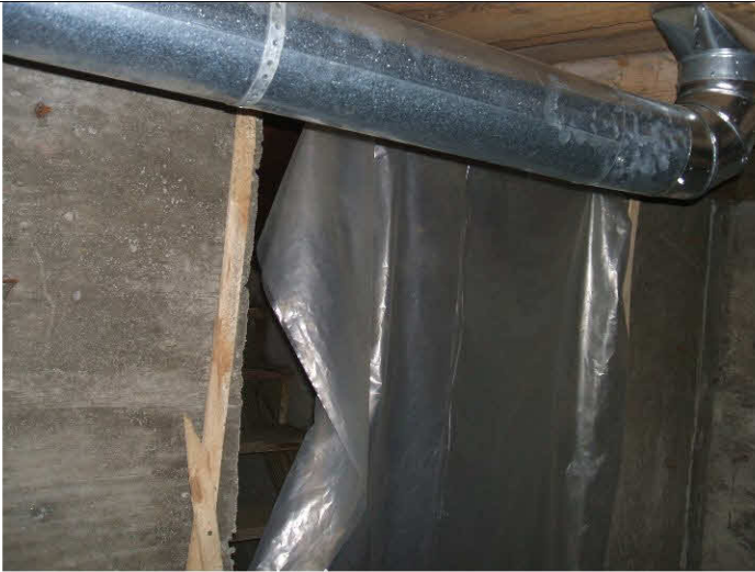
The basement bulkhead allows outside air into the basement.
