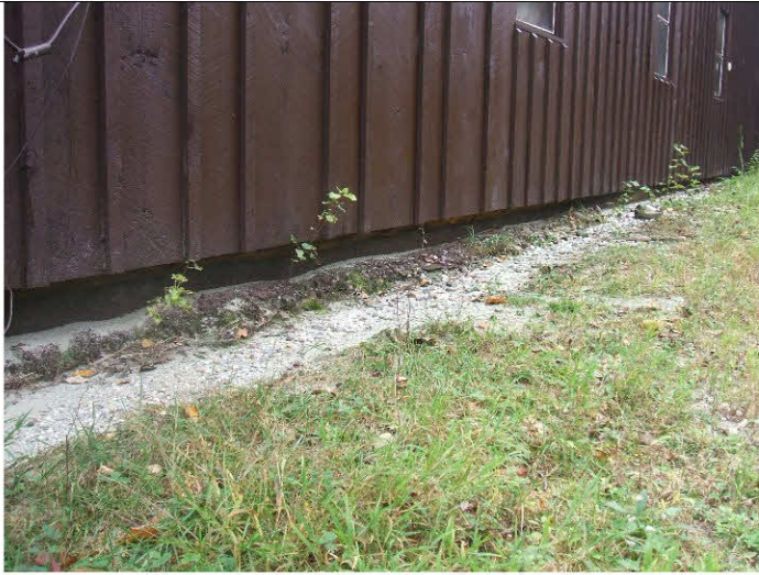
The exposed slab edge radiates heat to the outside and should be insulated like the rest of the wall.
