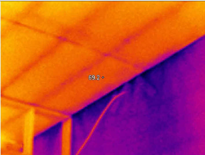
Air leakage at the wall to ceiling connection on an end wall.
