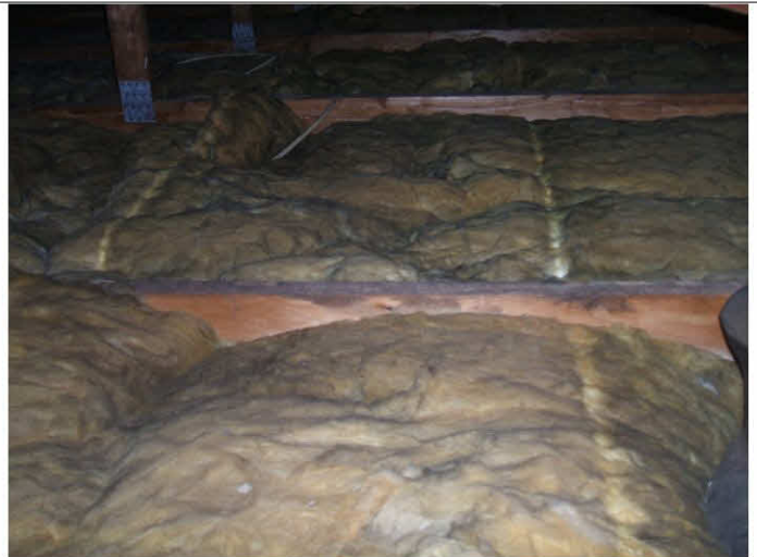
The lines are water lines below the roof purlins.
