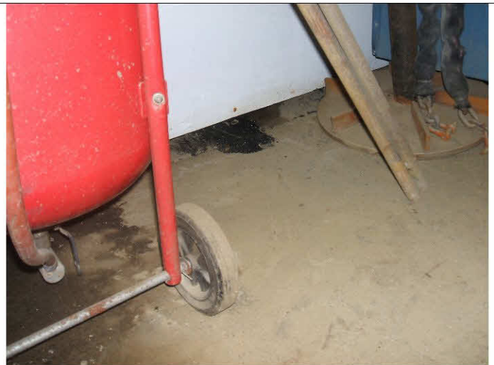
4" air space at the bottom of the wall where cold air pours in
