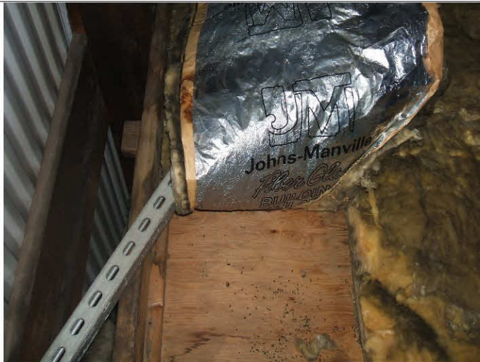
IR014987.IS2- Infrared image of the attic hatch and leaky wall to ceiling connection. 9/16/2010 6:18:25 AM
