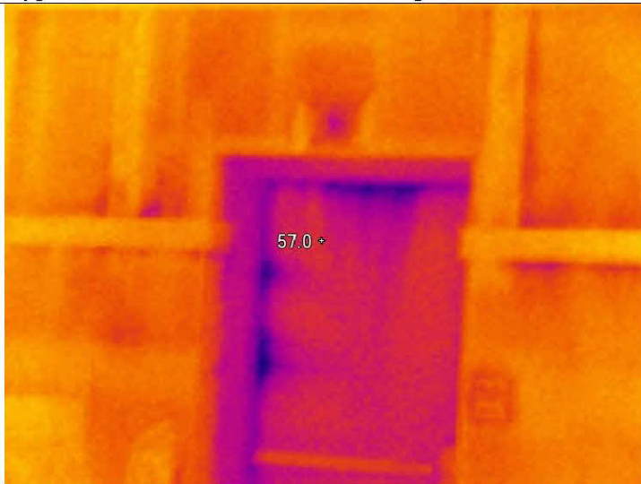
The door to the emergency stairwell door showing air leakage. This might be viewed as an “interior” door.
