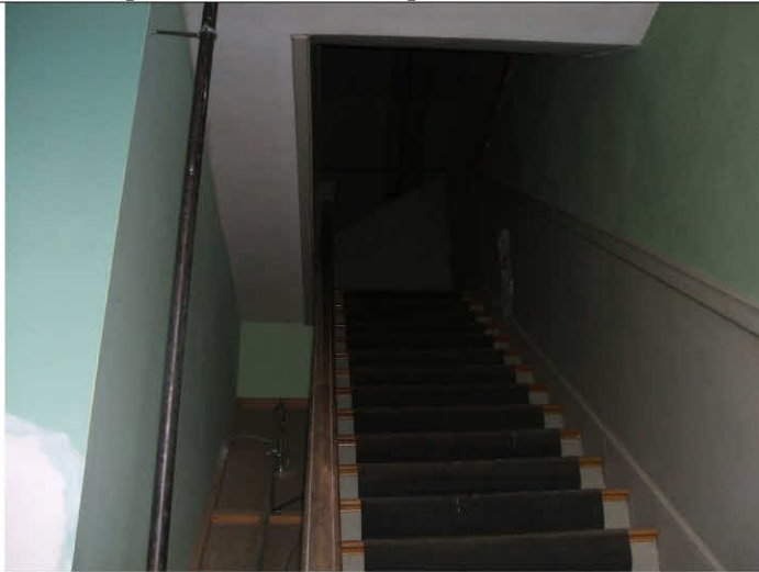
The hallway to attic needs to be separated from the heated space that surrounds it. The easiest way to do this may be to install an insulated and weather stripped door where the stairs pass through the flat ceiling rather than to try to insulate the walls and stairs.
