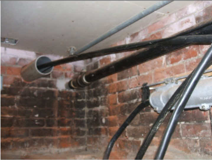
Basement conduit that is open to the outside. This is at the front of the building.
