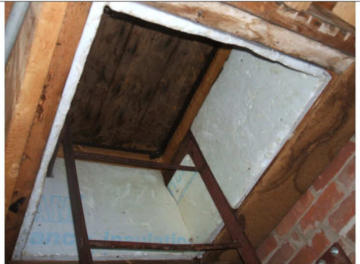
The stage ceiling hatch is not weather-stripped or insulated.
