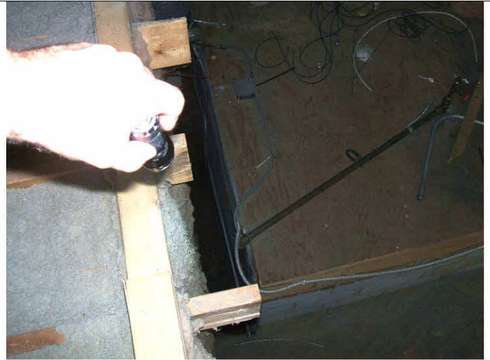
The elevator shaft is not insulated at the top and sides in the cold attic.
