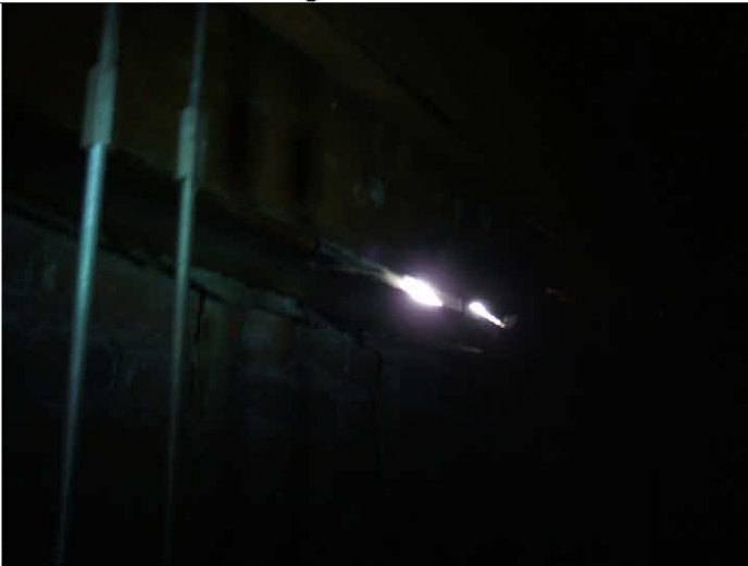
The stage ceiling has an air leak that can easily be seen from the stage. This should be sealed as part of an insulation scope for the whole ceiling and walls
