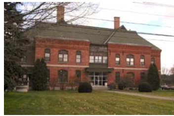
Hartford Municipal Building (in 100-Year Floodplain)
