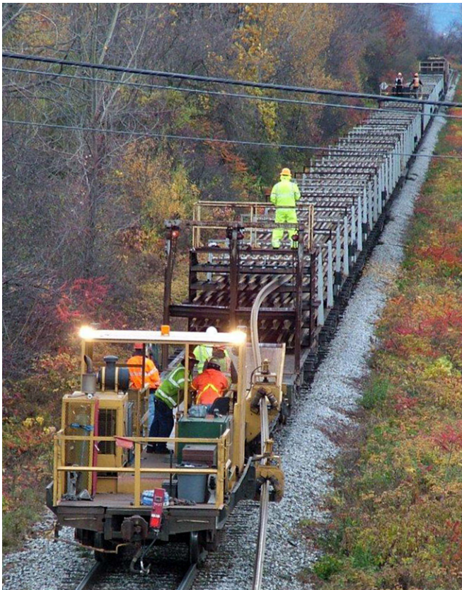
Continuously welded rail is being installed in Vermont as part of a nearly $80 million investment to upgrade rail in the Vermont.
