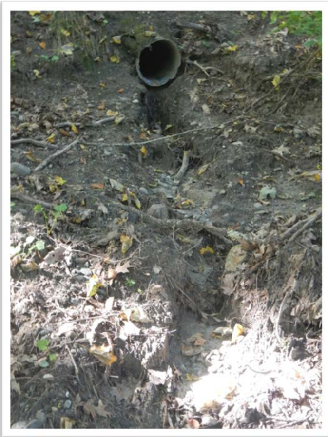
An eroded outlet on Carpenter Road Photo by Rita Seto, TRORC
