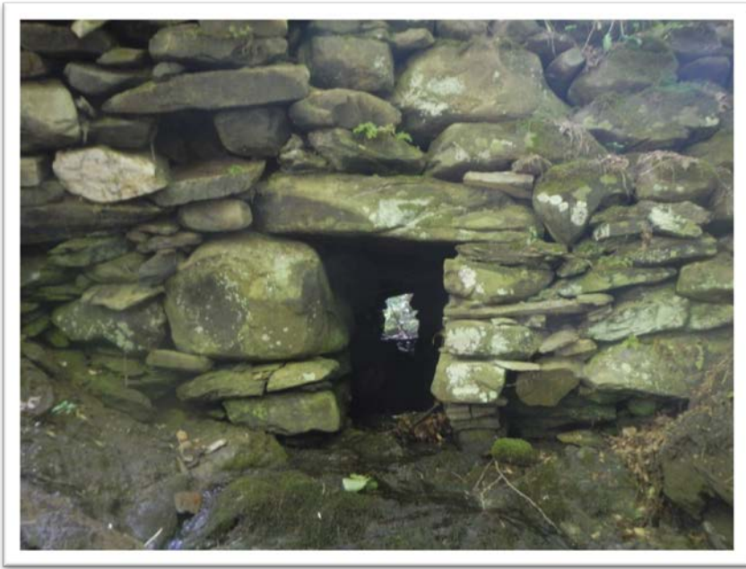
Old stone culvert on Brothers Road. Photo by Britta McOmber, TRORC
