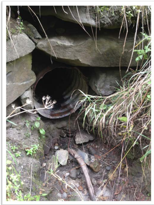
Rusted and perched culvert on Strafford Road. Photo by Rita Seto, TRORC
