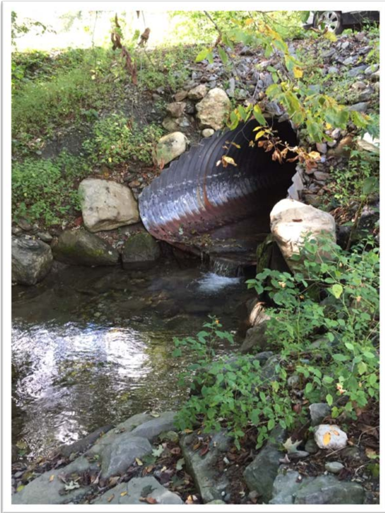
Perched culvert outlet on River Brook Drive Photo by Rita Seto, TRORC
