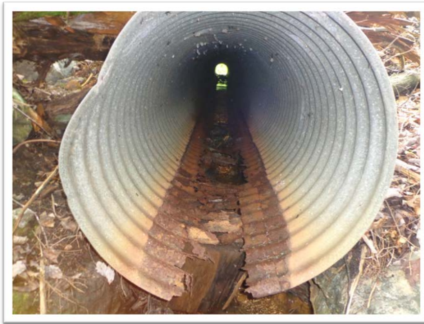
Rusted culvert on Lookout Road. Photo by Britta McOmber, TRORC
