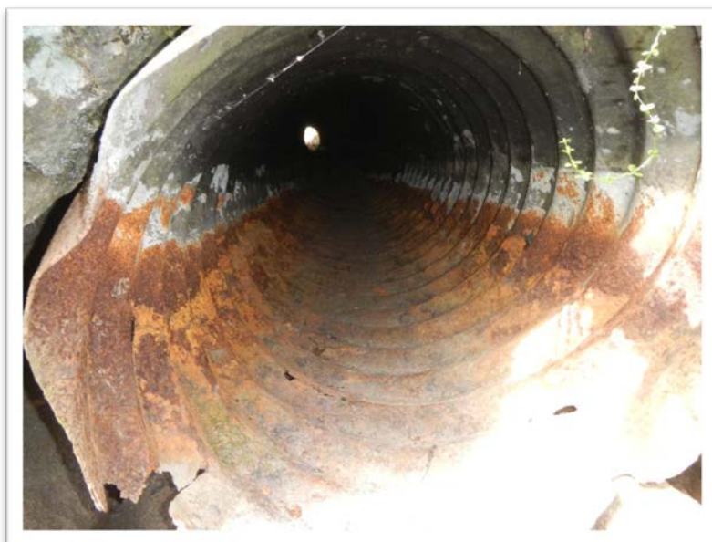
A rusted and crushed culvert on Happy Valley Road Photo by Rita Seto, TRORC
