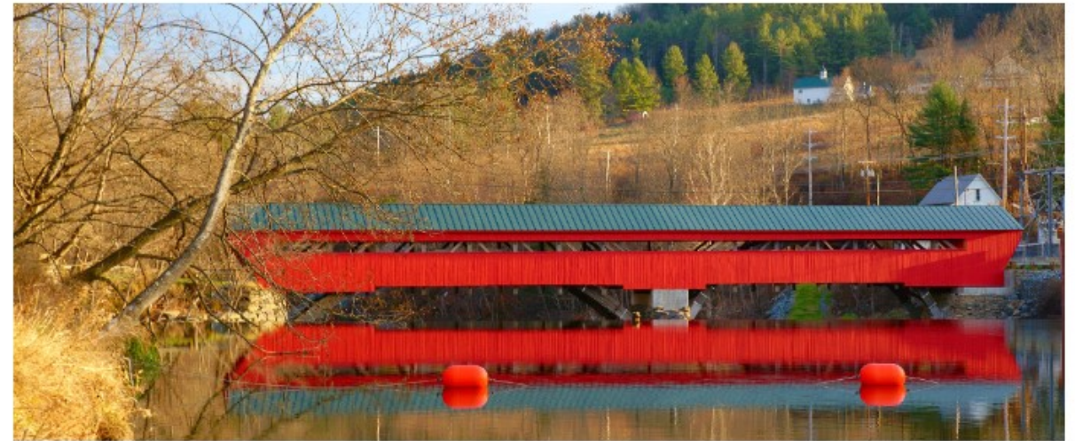
Tafstville Bridge | ©John Knox
