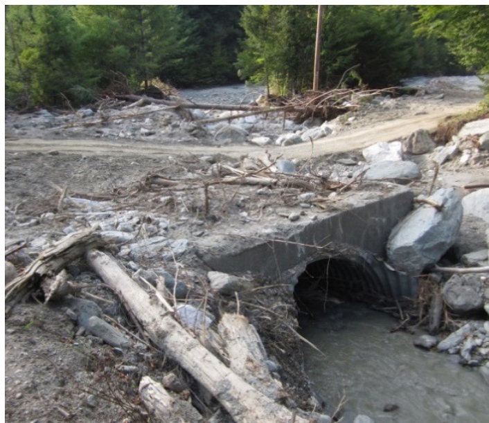
Severely Damaged Culvert, Stockbridge
