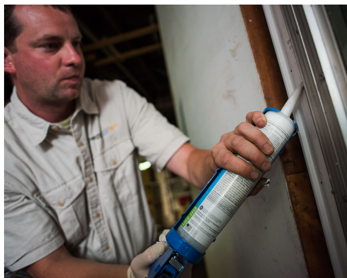
Air sealing a window frame with caulk Photo Credit: Capstone Community Action
