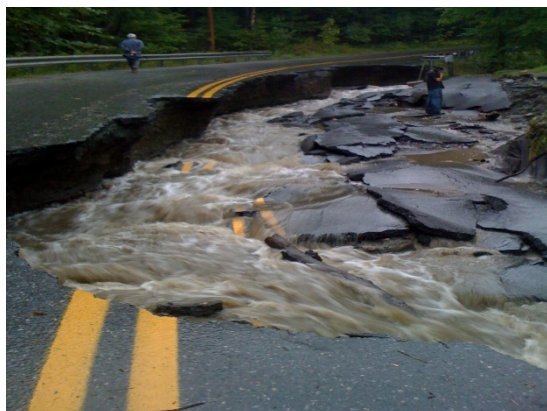
Road failure during storm
