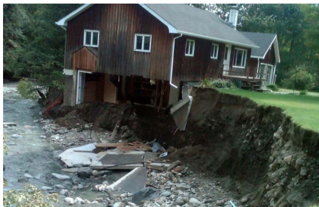
House undermined by lateral erosion from Irene
