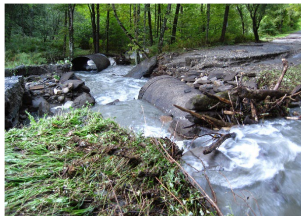
Culvert Washout during Hurricane Irene, Lower Lime Pond Road. Photo courtesy of Gina Lancaster.
