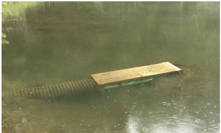
Beaver Baffle installed in Barnard (2017), Photo from VT ANR Natural Resources Atlas
