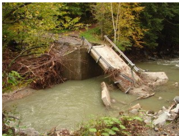
Bridge collapse on Route 12 North during Irene. Photo courtesy of Gina Lancaster.
