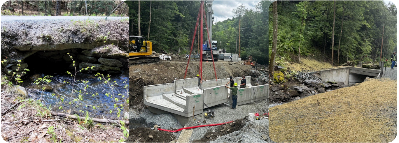
Undersized culvert replacement - Jenneville Road, Hartland, VT
