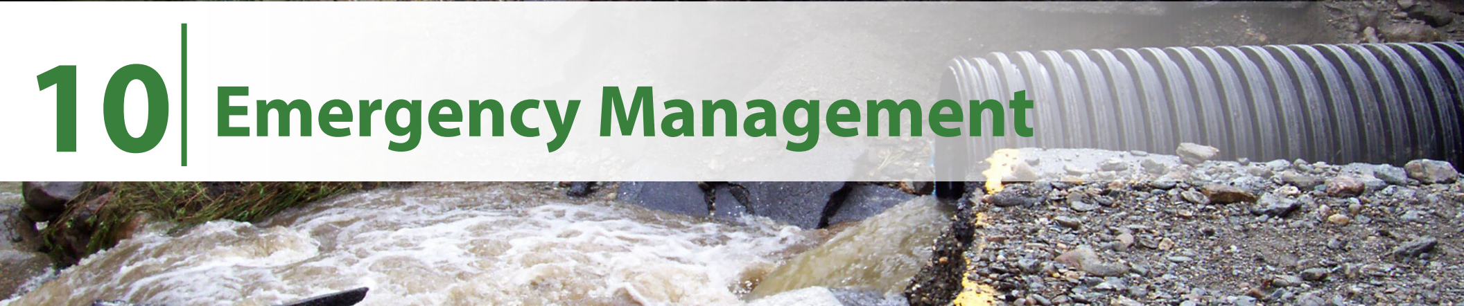
Route 125 Flooding | Source: TRORC
